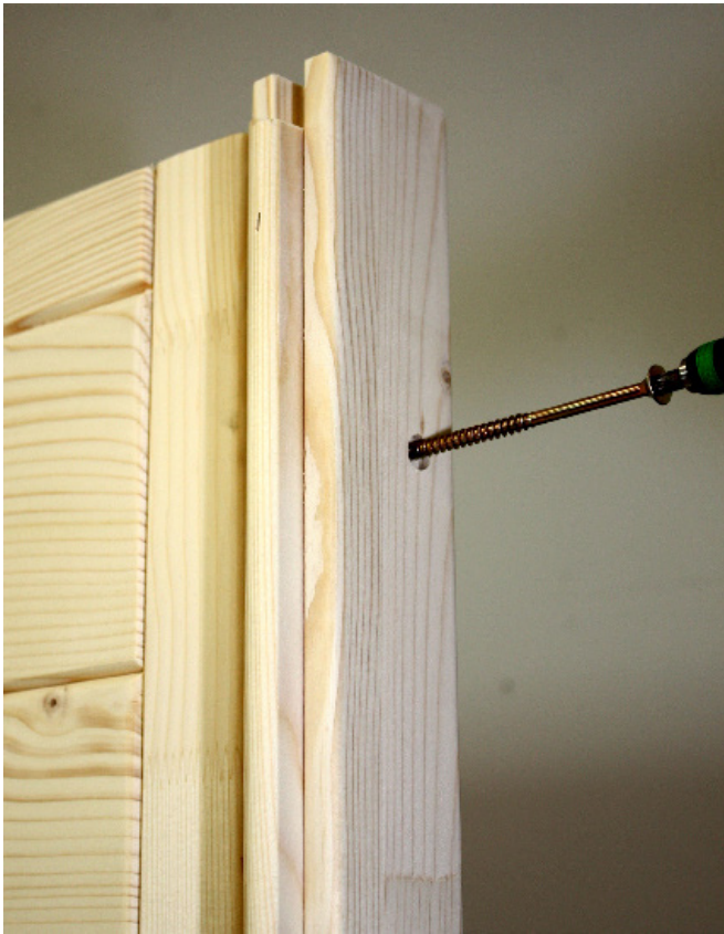
8 screws 6 x 120 mm per corner post
