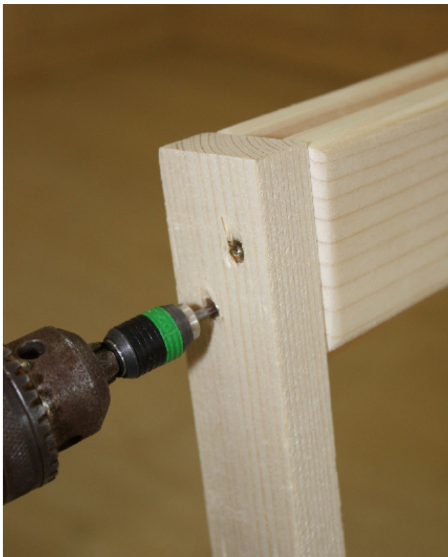
Remove transport strip from the door frame
