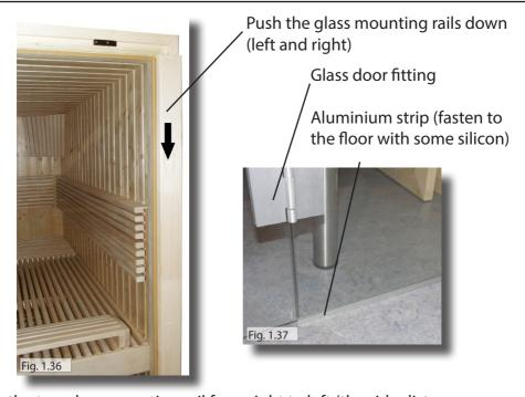
Push the top glass mounting rail from right to left (the side distance on the left and right should be the same)
